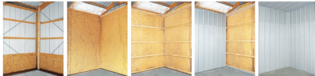
View of corner section before insulation
